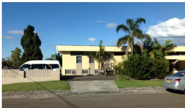
Western elevation of the hospital near the north-west corner
