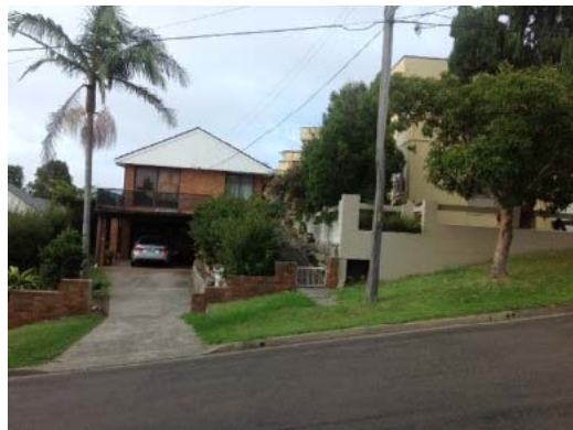
North-east corner & adjoining No.182 Wyndora Ave
