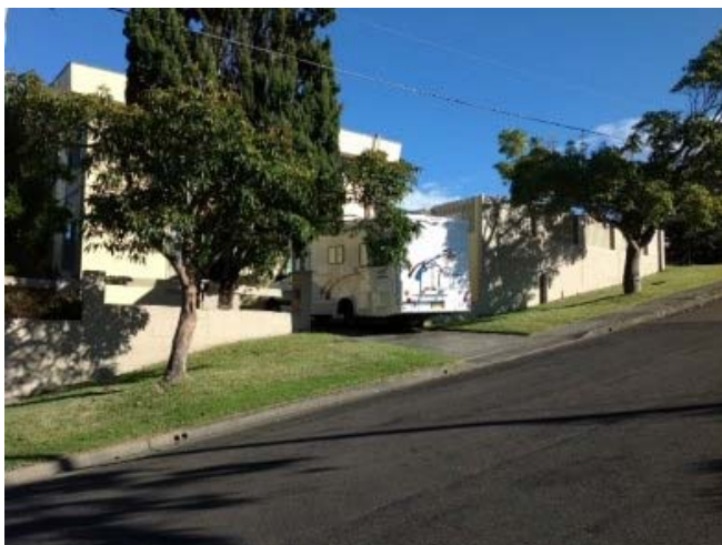
Northern elevation of the hospital
