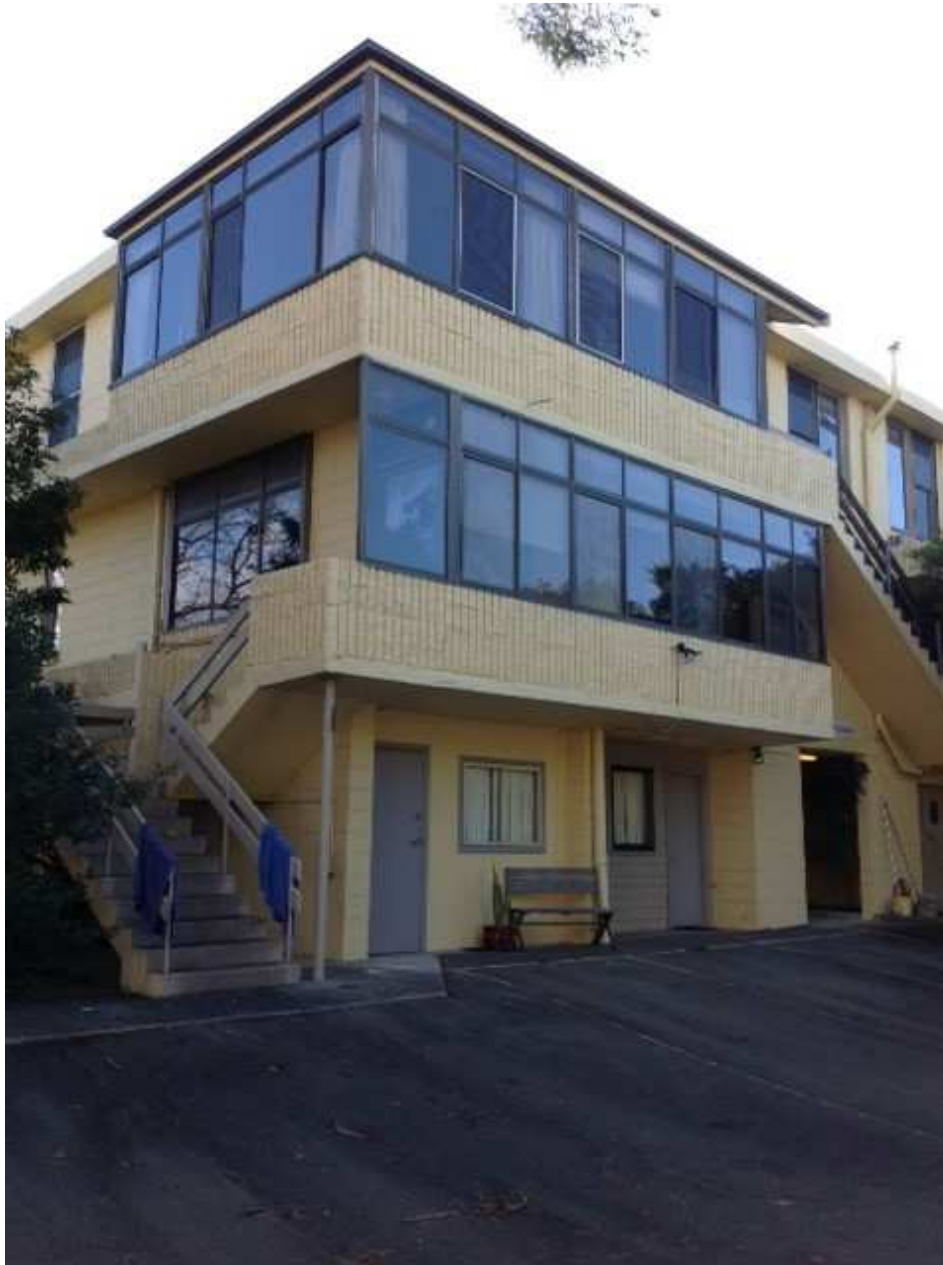
Figure 3 – Existing building and (disused) car park
