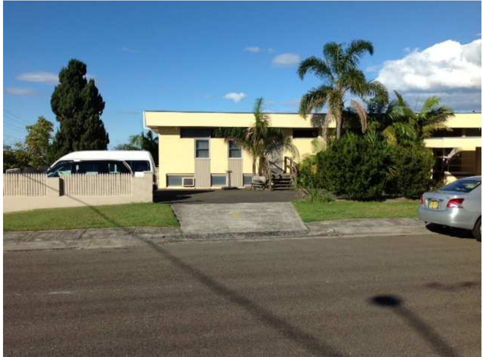
Figure 4 – Existing building and site entrance
